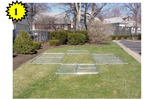
1 Lay all panels flat on ground
