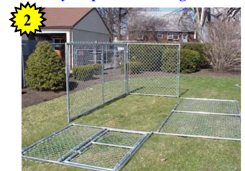
2 Attach two clamps for each corner
